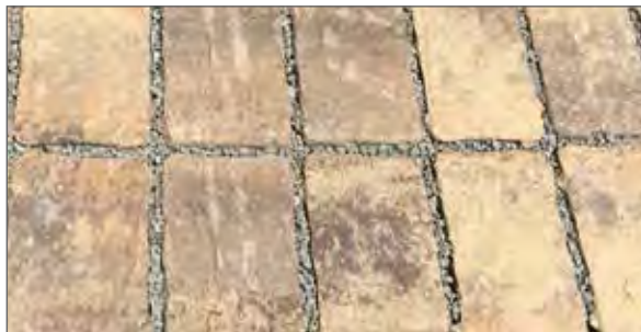
Exhibit 3.45: Permeable Pavers Median
