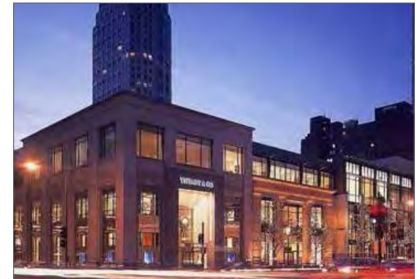
Exhibit 4.14: Low-Rise Commercial Building Example
