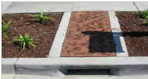
Exhibit 3.70: Treewell Filter - Stormwater Treatment
